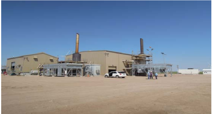
Compressor Buildings and Engine Exhaust
