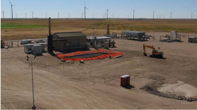
Start of the Second Compressor Foundation
