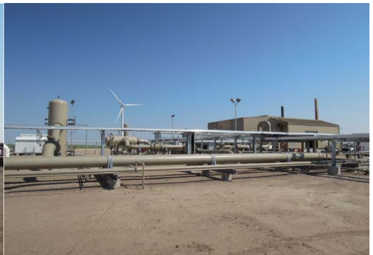
View of the new surface facilities
