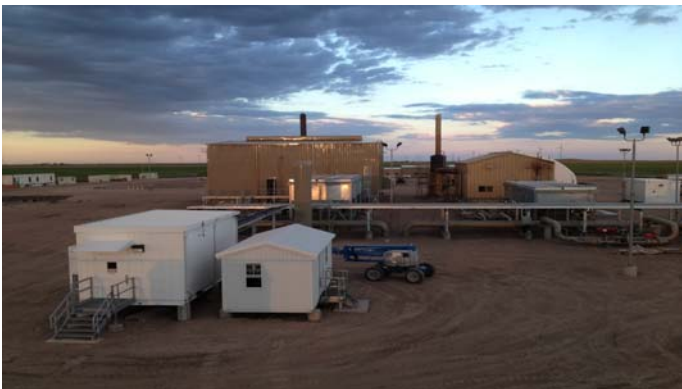
New Buildings and pipe racks
