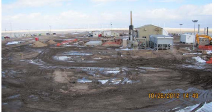
The challenges of Fall Construction!!!
