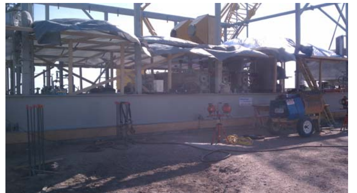
Working on our first compressor skid
