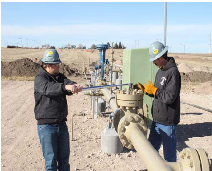
Tightening a check valve cap
