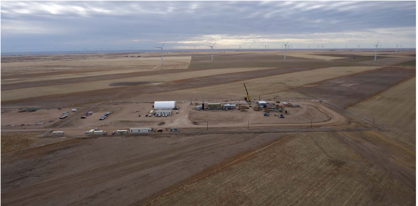
View of ECGS Construction from an On-Site Wind Turbine
