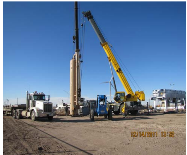
Contacter Tower Being Set
